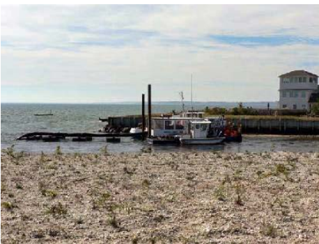
Dredge working in Cedar Beach Inlet
